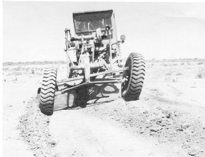
Fig. 4. Dike construction using a motor grader. The dike is being constructed from the lower side.
