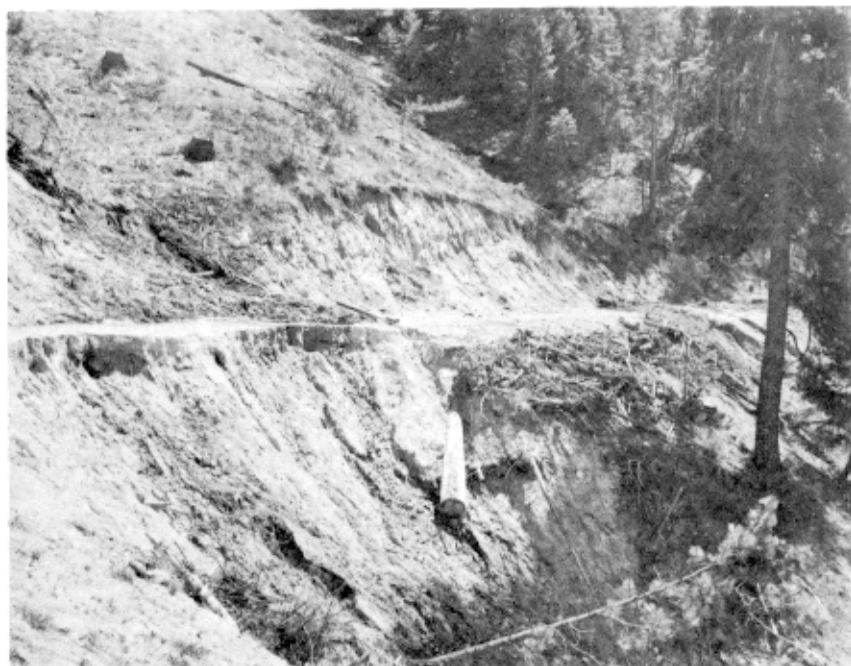
Fig. 1. On extremely adverse sites, roadways must be stabilized by planting.
