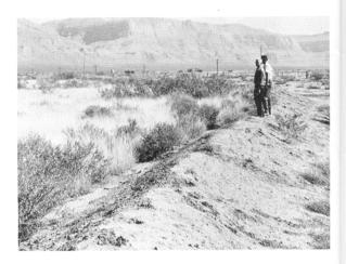
A waterspreading scheme on the Prather Ranch, south of Alamogordo. Wild water on rangeland can often be used to increase forage production and substantially reduce erosion.
