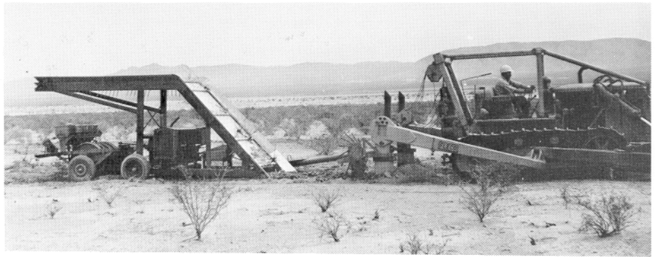
Fig. 1. First model of overhead conveyor being pulled behind a D-7 tractor and a rootplow.
