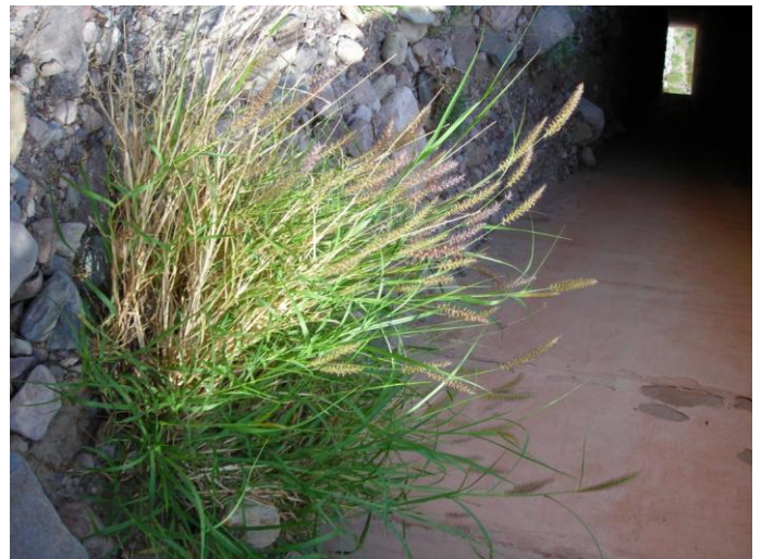
Photo 4. Buffelgrass clump along a culvert in Big Bend National Park.
