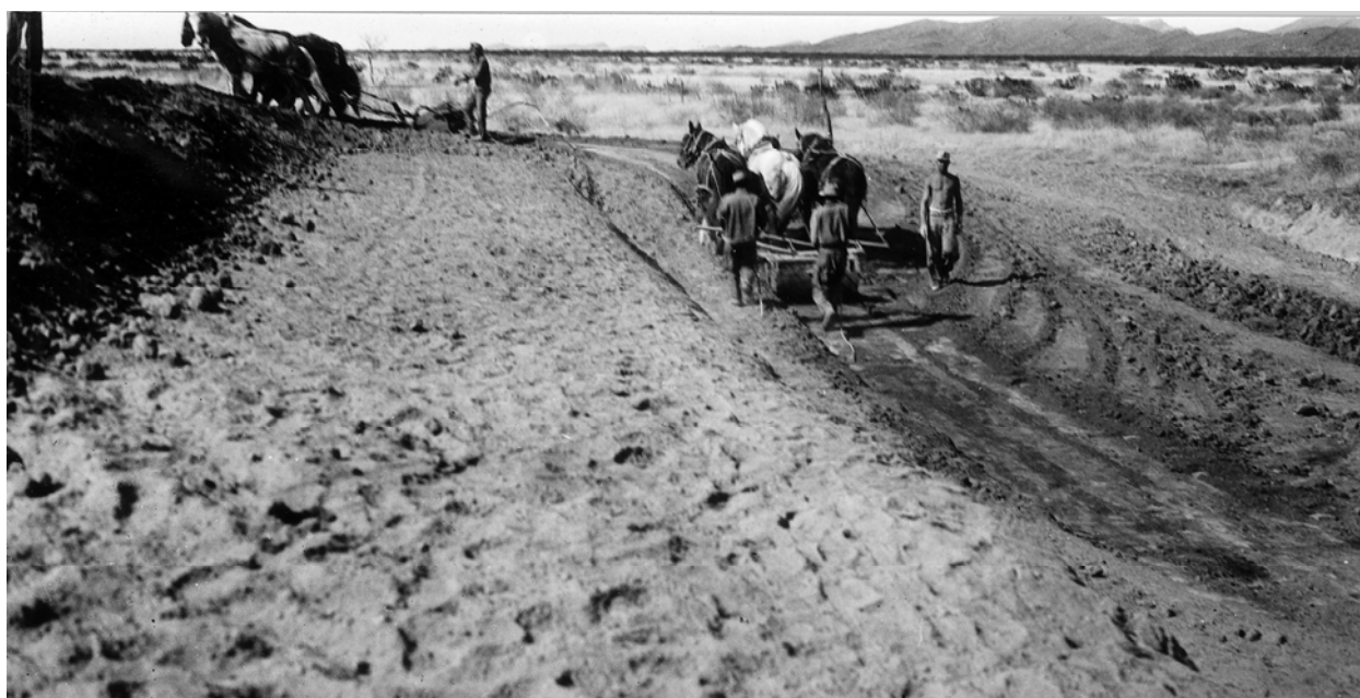
Figure 6. Big Meadows stock tank being built by Civilian Conservation Corps at the Jornada Experimental Range on 3 April 1934 using three-horse Fresno teams.
