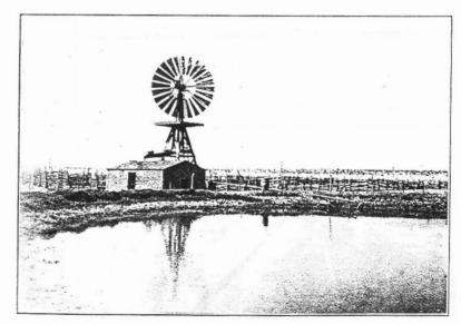
FIG. 2.—A PUMPING PLANT AND RESERVOIR IN NEW MEXICO, THE WELL IN CONNECTION THEREWITH BEING 330 FEET DEEP.
