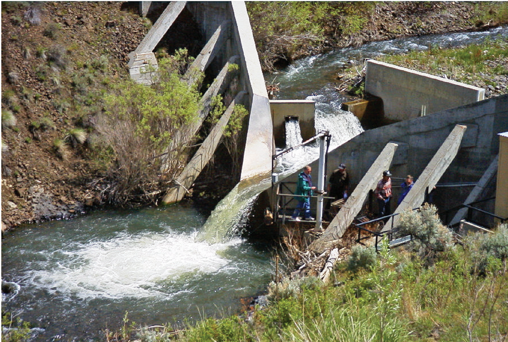
Figure A1-65. Reynolds Creek Experimental Watershed (RCE USFS) is located in southwestern Idaho and includes Great Basin rangeland at low elevations with aspen and Douglas fir communities at higher elevations. Streamflow is measured using a drop-box weir. (Photo from RCE photo gallery.)
